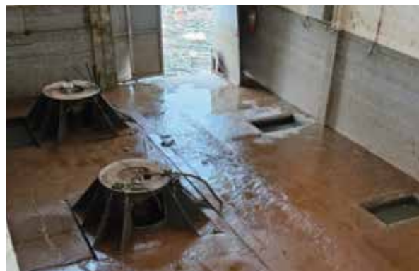
Motors were moved to prevent damage, making the station inoperative.
