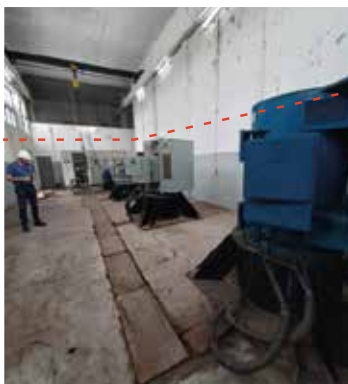
Water level inside pump station during the floods.
