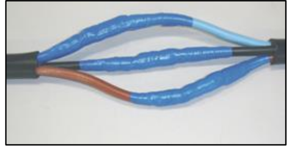
Figure 25 – Splicing step 5
