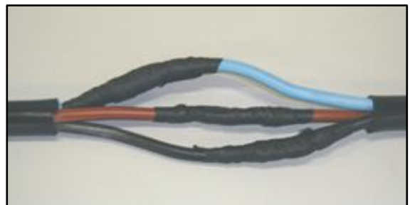
Figure 24 – Splicing step 4
