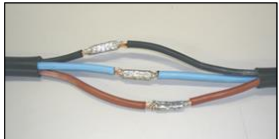
Figure 23 – Splicing step 3
