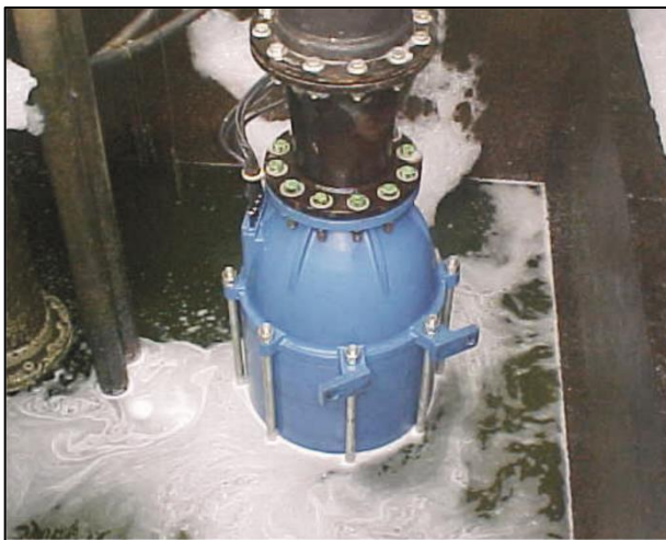
Figure 2 – Amphibious Pump in a Tank
